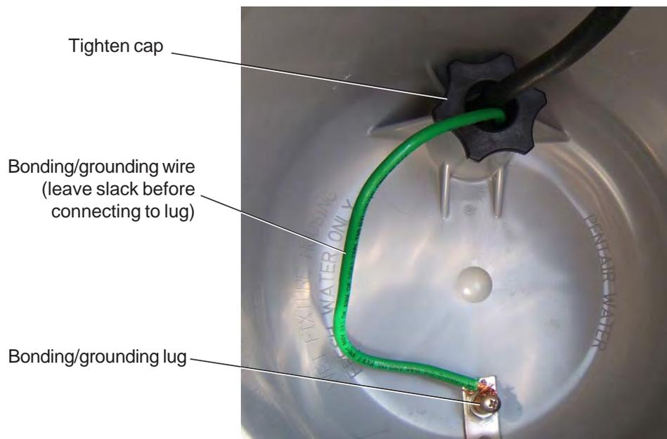
14. The niche installation is complete. The niche is ready for the light installation.
